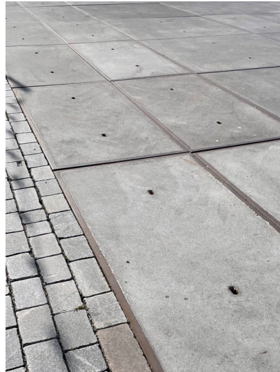
Prefab betonplaten i.c.m. kinderkopjes
