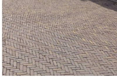
Bestrating in keperverband
